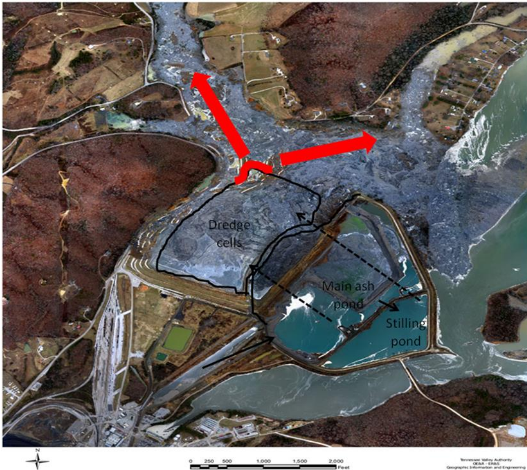
Aerial Image Of Kingston Ash Slide 12/23/08
