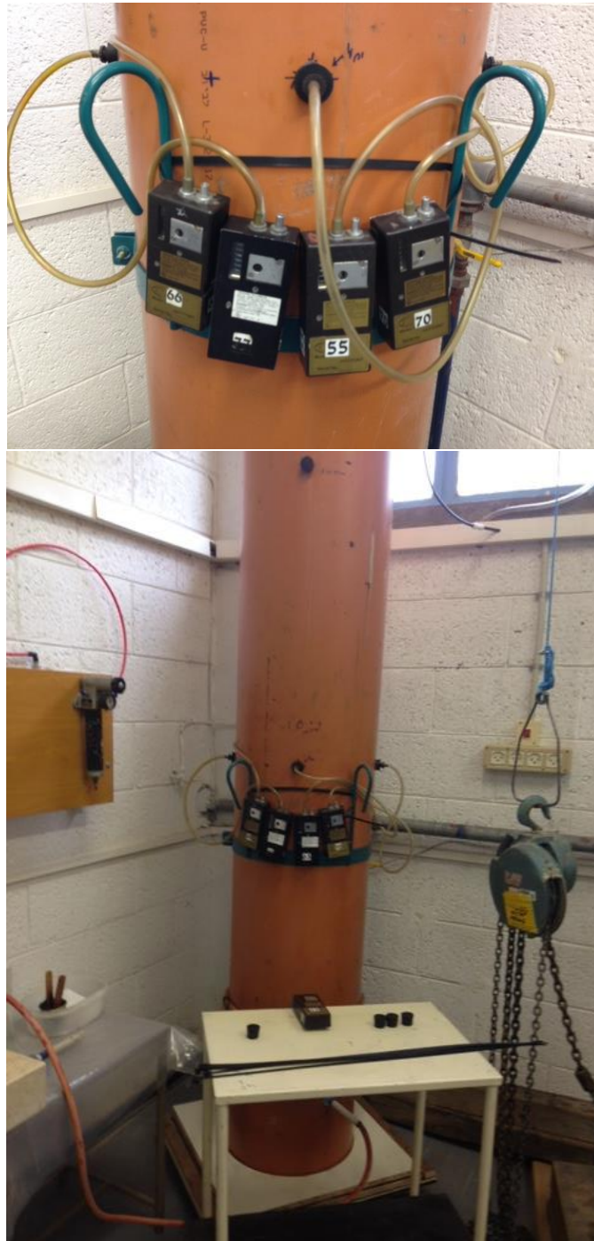
Figure 4: Ammonia monitoring systems mounted on the column
